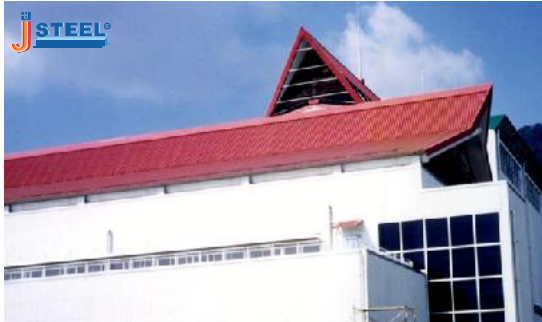
Wayang Windu Power Plant - Bandung
